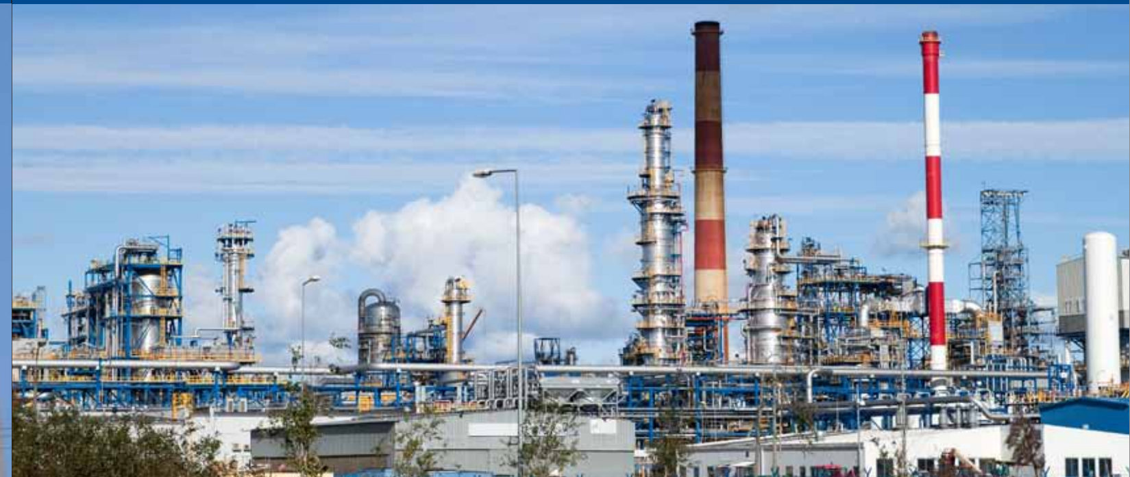
Petro Chemical Plant
